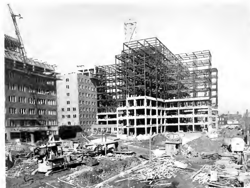
Advances in design and construction of highways, bridges, hospitals, and public buildings are credited to engineers in the career civil service. The modern hospital pictured under construction is one of a number of major construction projects designed by Federal engineers.
